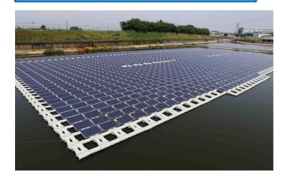
• Total cost of FPV sightly higher (10-15%) than ground-mounted, but nearing price equivalence
