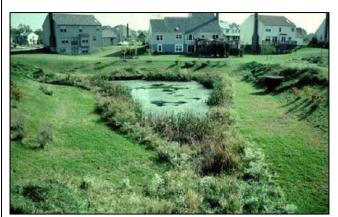
An Extended Detention (ED) Pond relies on 12 to 24 hour detention of stormwater runoff after each rain event. An under-sized outlet structure restricts stormwater flow so it backs up and is stored within the basin. The temporary ponding enables particulate pollutants to settle out and reduces the maximum peak discharge to the downstream channel, thereby reducing the effective shear stress on banks of the
