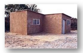
Casa Grande estimates a home constructed using Grancrete ® costs approximately \$6,000 (USD) for labor and materials. It is estimated that an 800 SF home could be constructed for \$10,000 (USD). According to Casa Grande, typical apartments in Bombay, India are 400 SF. It is hoped that international organizations will subsidize mass scale production globally using the product (ANL, 2005).
