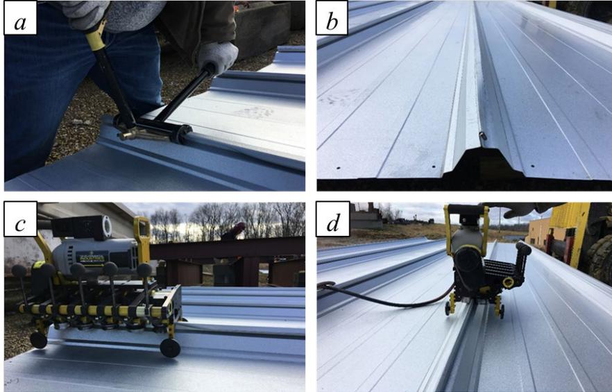
Figure 8 Pictures showing the seaming process in sequential order
