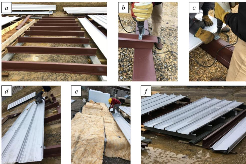
Figure 7 Specimen construction process
