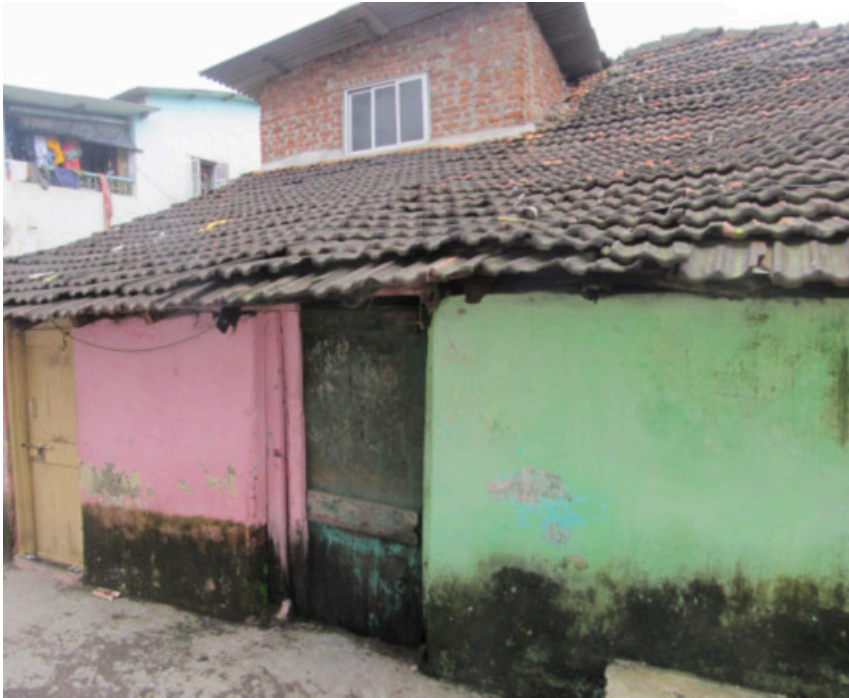
Figure 17: Most buildings in the settlement are built out of a mixture of building materials and construction techniques. In the house pictured here, one can distinguish the recent additions because of the different construction materials.
